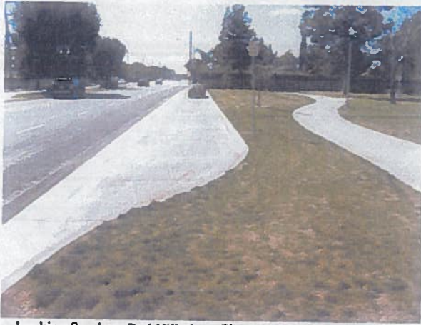
Looking South on Red Hill along Pine Tree Park Frontage
