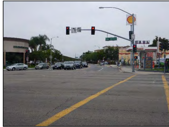
Wide signalized intersections
