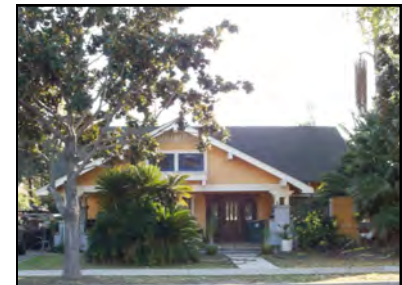
An example of a gable roof with exposed roof beams and elongated rafter ends at 400 West Main Street.
