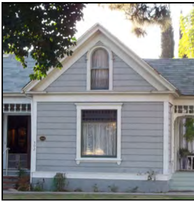
Pediment Gable at 302 A Street
