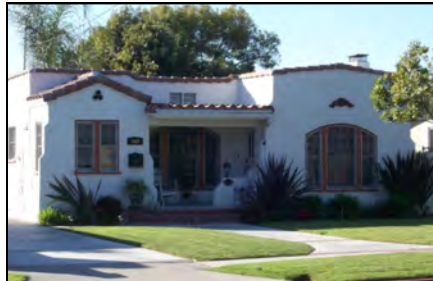
Turner House 160 South Pacific Street 1927 Spanish Colonial Revival (Mills Act Property)
