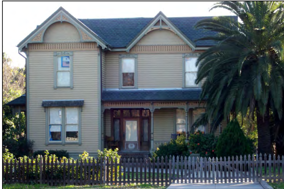
420 West Main Street Vance House
