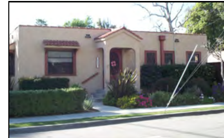
Slusser House 705 West Main Street 1926 Spanish Colonial Revival
