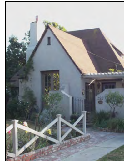
320 West 3rd Street Holmes House (Tudor)
