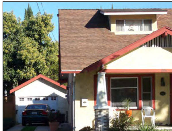
The Fewell House, at 155 Pacific Street, has good architectural compatibility, especially with the detail just under the pitch of the roof.
