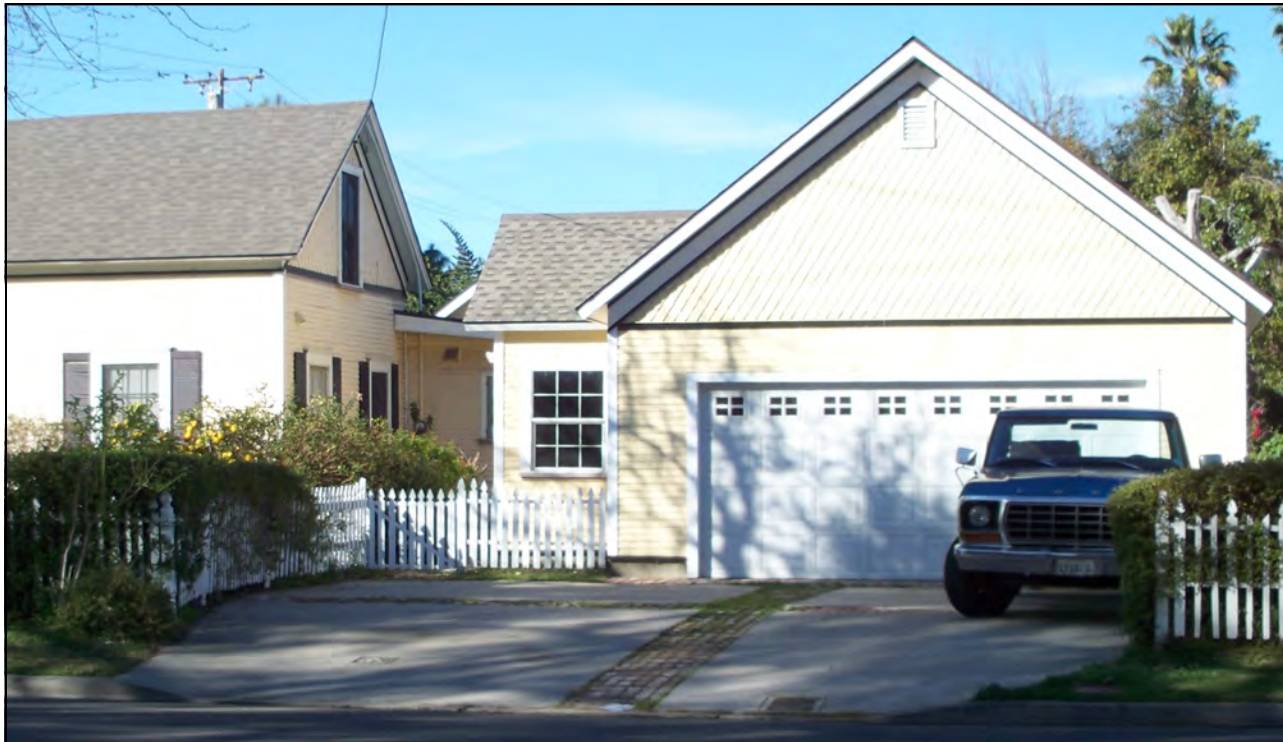
Appropriate accessory building and garage at 265 South Pacific Street, Brown House.
