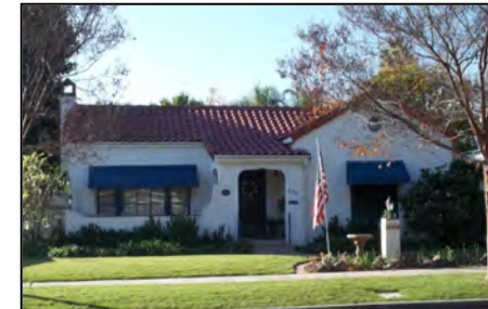
Carter House 250 Pacific Street 1928 Spanish Colonial Revival
