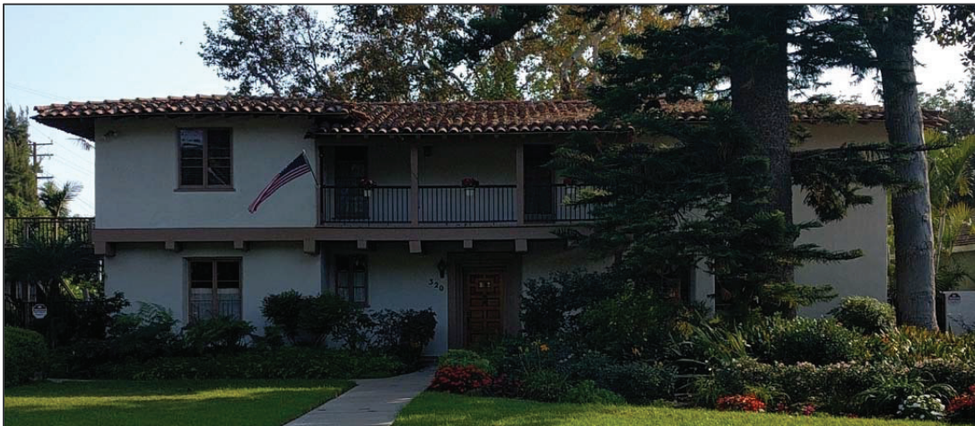
Pankey House (320 W. Main Street, 1928). ARG, 2021.
