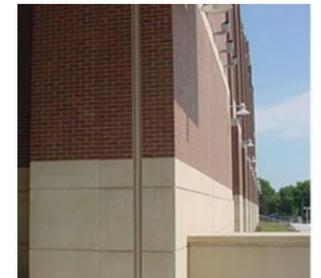
*Regularly spaced expansion joints form patterns on the building facade.*
