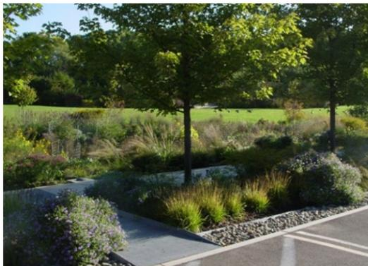
*Landscaping shall be designed to provide biofiltration and bioretention functions.*
